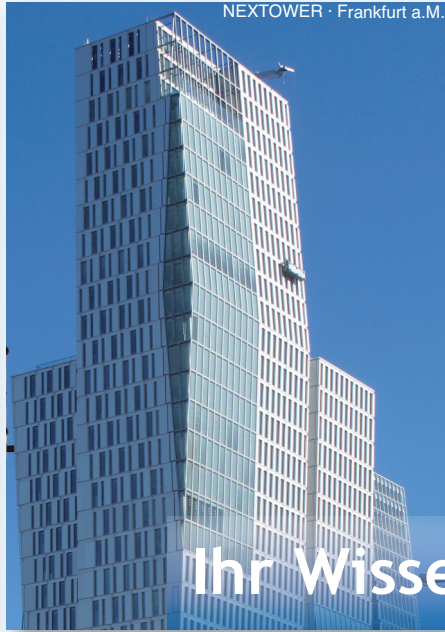
NEXTOWER · Frankfurt a.M.
